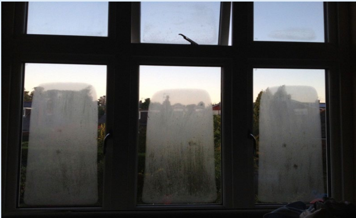
Fig 1 – External condensation (border effect and pad residue on A Rated DGU Installation).
